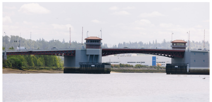
PHOTO CREDIT: KING COUNTY WASTEWATER TREATMENT DIVISION
