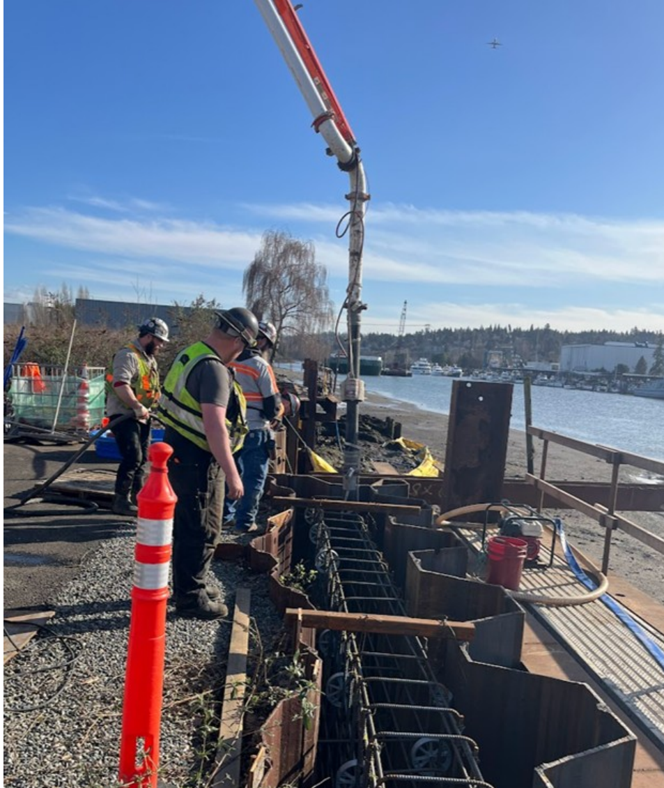
Filling the space between the original and new SMA 9 bulkhead wall system (sheet pile wall) with concrete (Geosyntec Consultants, week of March 3, 2025).
