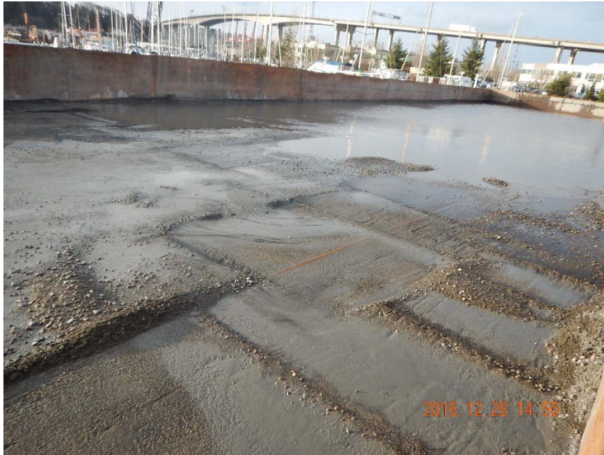
Photo 2-A: KP-2 after the GS+AC placement was complete.
