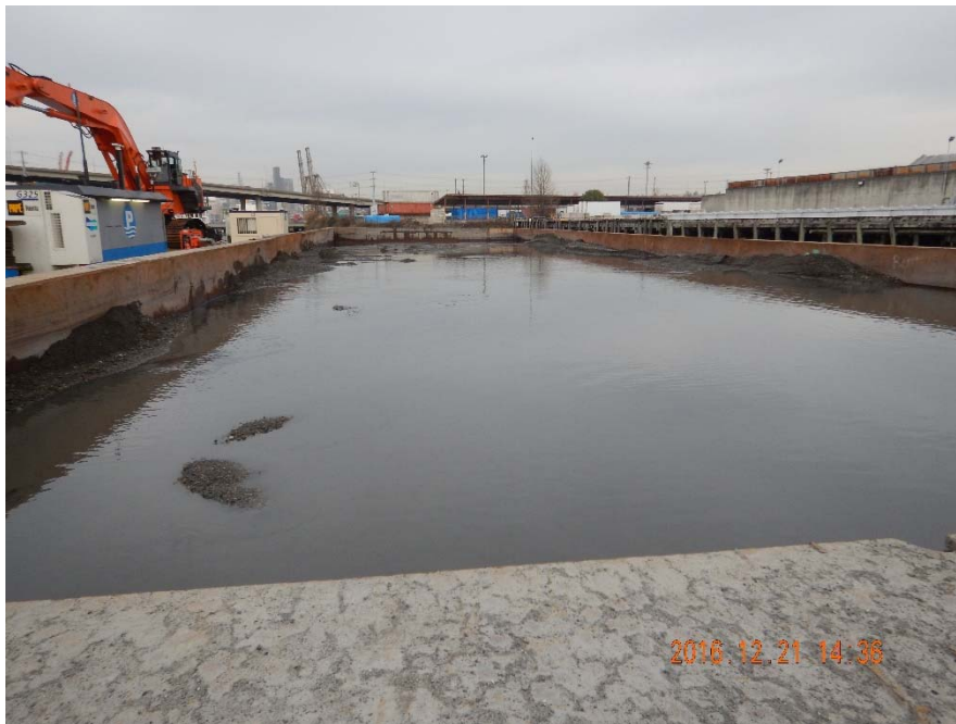
Photo 1-B: GS+AC barge after the material was spread out to submerge.
