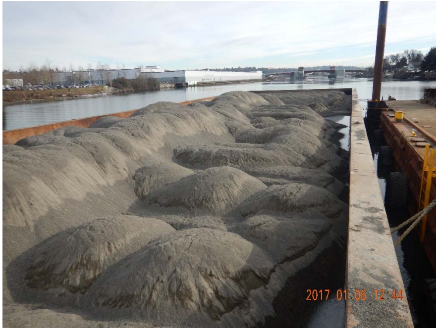
Photo 2-A: Sand+AC ENR material prior to levelling and soaking.
